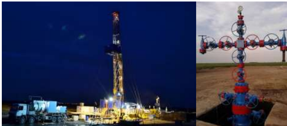
Figure 3 - Jimbolia-100 Well - wellsite (night view), Xmas tree
